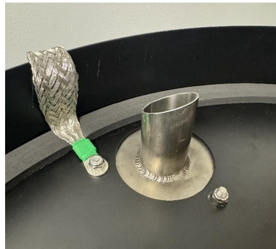
Figure 4: Bottom View of Ground Strap Installation
